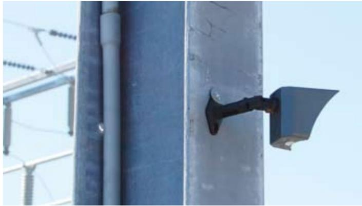
This is a close-up of the video monitor camera located inside the station and "looking" out toward the perimeter fence.
