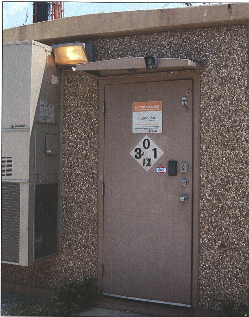
This view of a shelter shows the camera above the door and a proximity card reader on the door above the doorknob. The camera also views any approach to the air conditioner. Some thieves have removed air conditioners to gain entry to the building and have stolen all or part of the air conditioners for the metal they contain.
